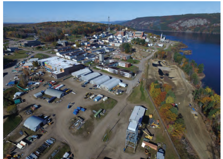
A significant investment is being made in the revitalization the Chalk River site infrastructure and facilities. CNL continues its legacy of cutting-edge science while adapting to the needs of its customers both federal and commercial. Above, Building 350, a new active materials science laboratory complex is scheduled to open this year.
