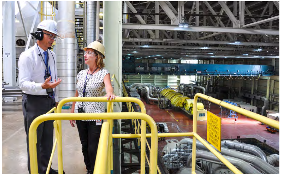
Since joining Bruce Power in 2016, Mike Rencheck has been connecting with stakeholders across the province. He's met with elected officials such as Parliamentary Secretary to the Minister of Natural Resources Kim Rudd (above), employees at town halls at both OPG and Bruce Power (cover page bottom) as well as organizations like CANDU Owners Group (cover top right), where he attended the December 2016 General Business Meeting.
