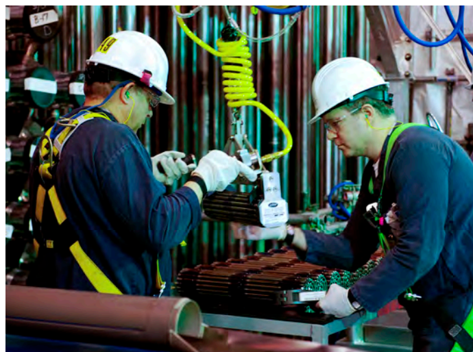
NB Power's Point Lepreau Station refuelling after refurbishment
